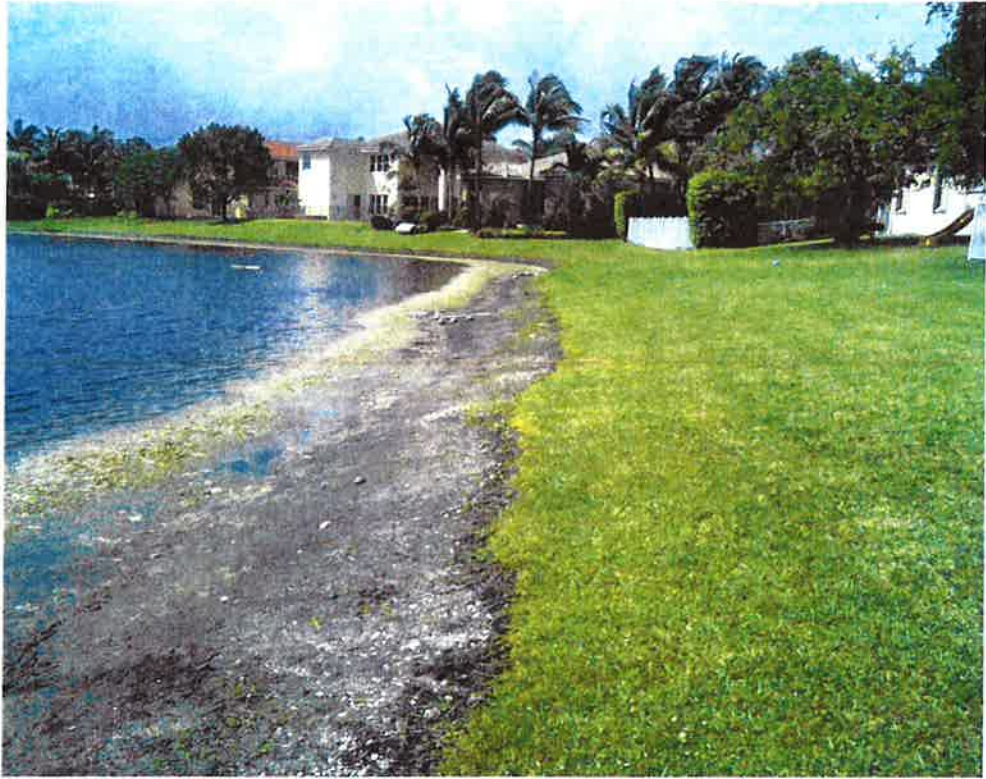
Figure 21 – South End of Lake 4 off Wilbur Way Looking North on 05/29/2015
