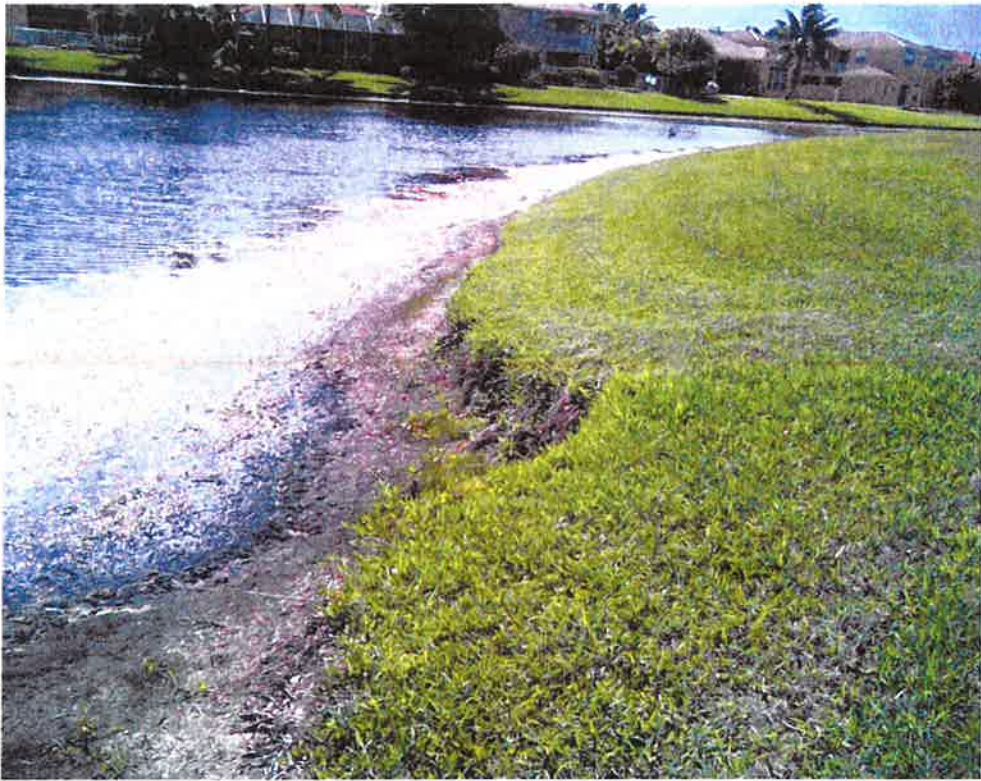
Figure 19 – South End of Lake 4 Looking East on 05/29/2015
