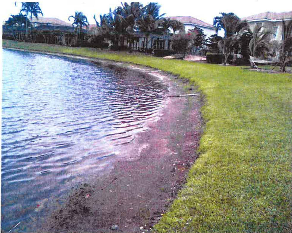
Figure 24 – West End of Lake 6 Looking South on 05/29/2015
