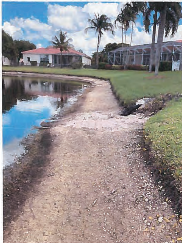
Figure 39 – 3-26 – Southeast corner of southwest finger of Lake 3. Erosion around pipes from residence.
