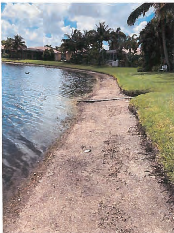
Figure 29 – 3-16 – South end of southwest finger of Lake 3; erosion noted at irrigation intake
