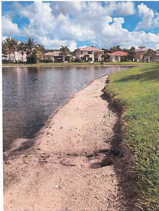
Figure 53 – 4-12 – Middle of south side of Lake 4; erosion in lake bank
