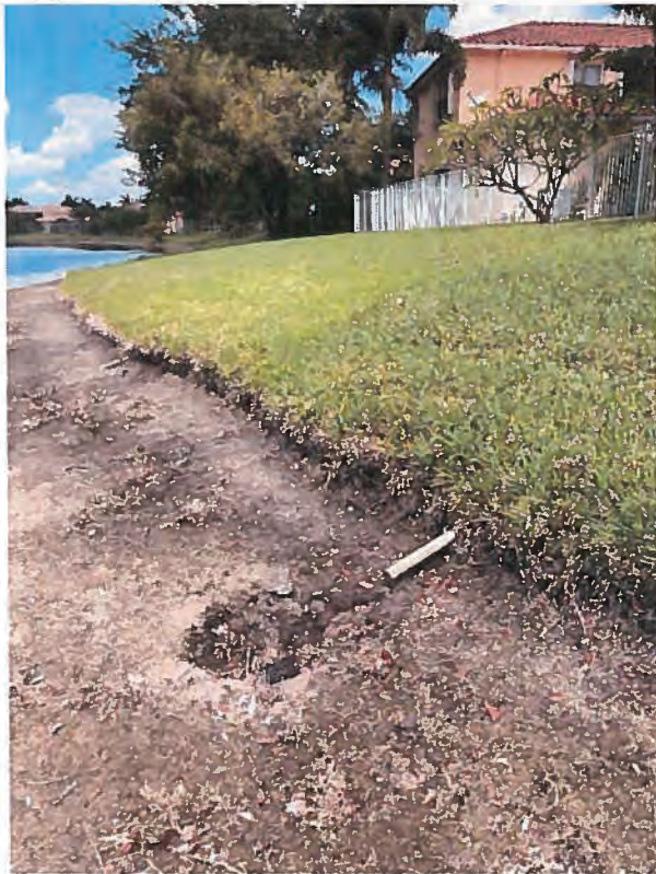
Figure 64 – 5-4 – North side of Lake 5; erosion from pipe drain
